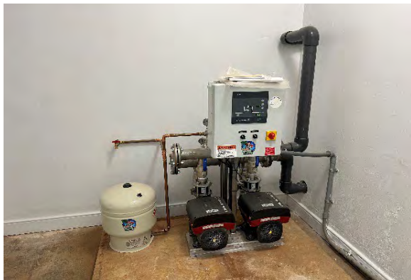
Admin. Bldg. Domestic Water Station and Plumbing
