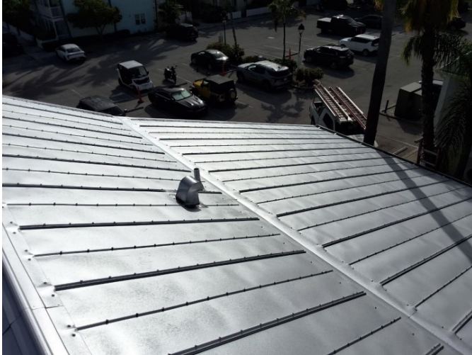
Metal roof photos
