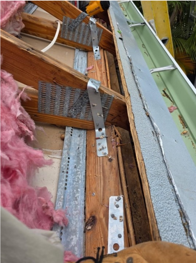
SWR SWR installed
