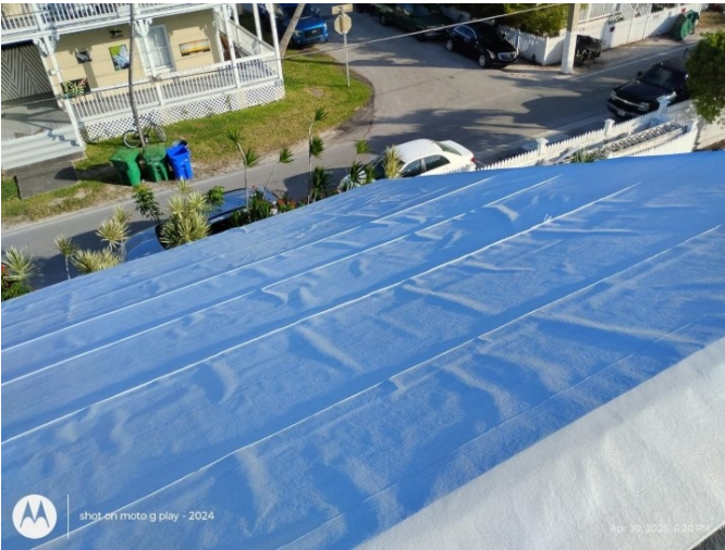
SWR SWR installed
