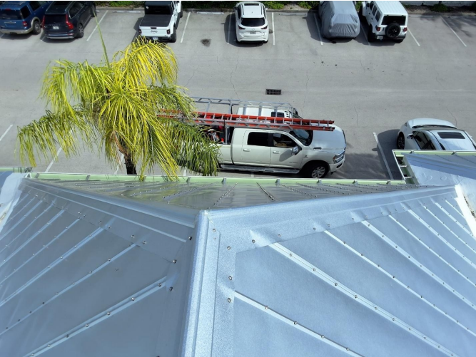
Metal roof photos
