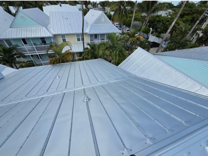
Metal roof photos
