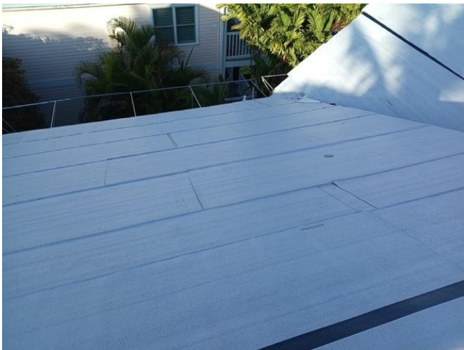
SWR SWR installed
