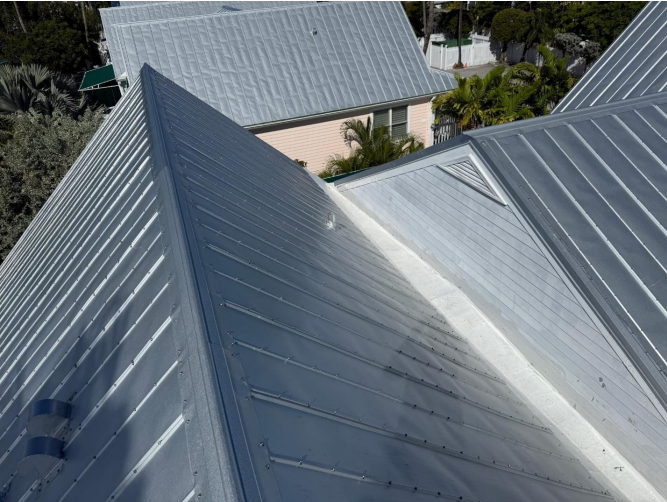
Metal roof photos
