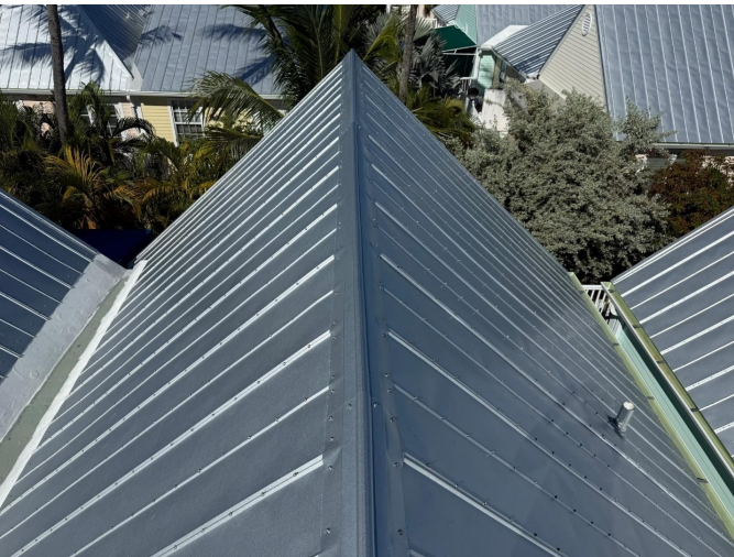
Metal roof photos
