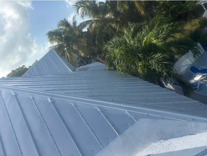
Metal roof photos
