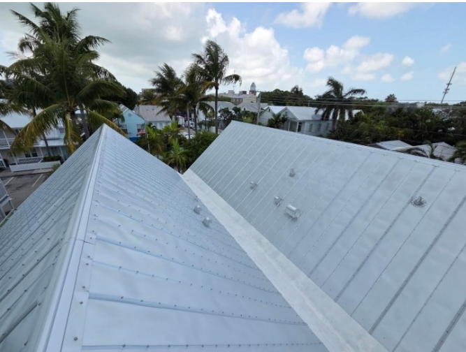
Metal roof photos
