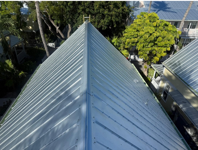
Metal roof photos
