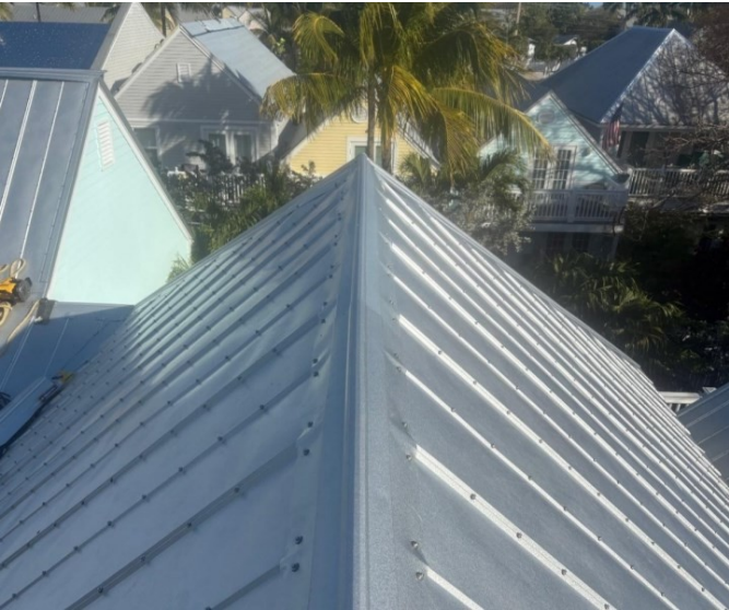
Metal roof photos
