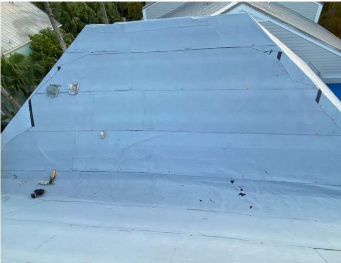
SWR SWR installed
