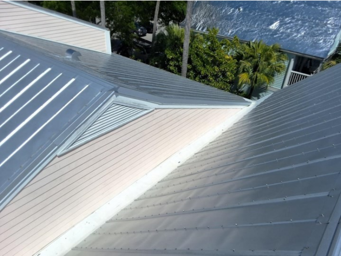
Metal roof photos
