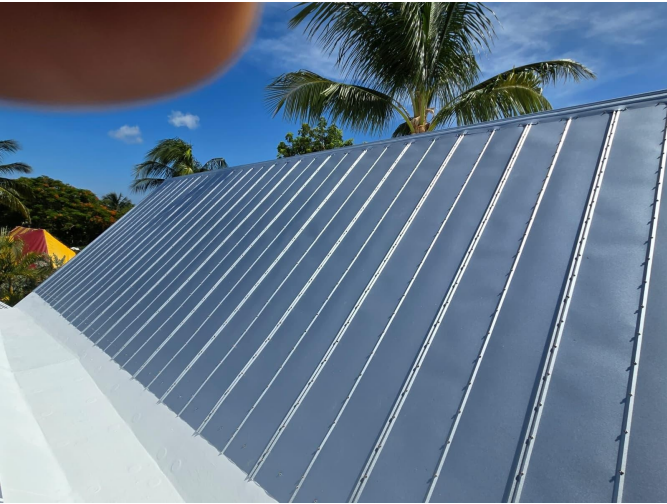
Metal roof photos
