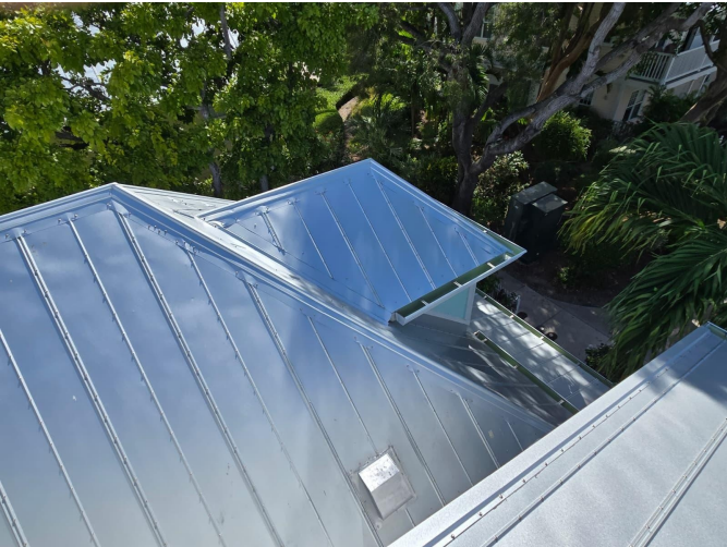
Metal roof photos
