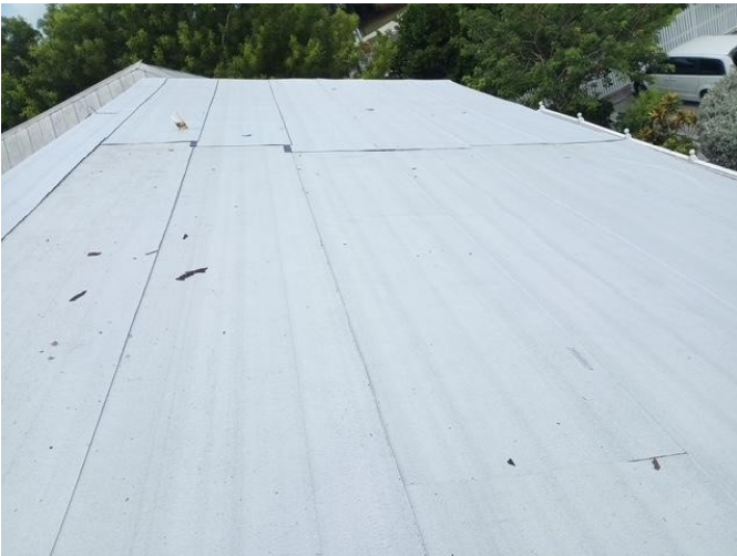
SWR SWR installed
