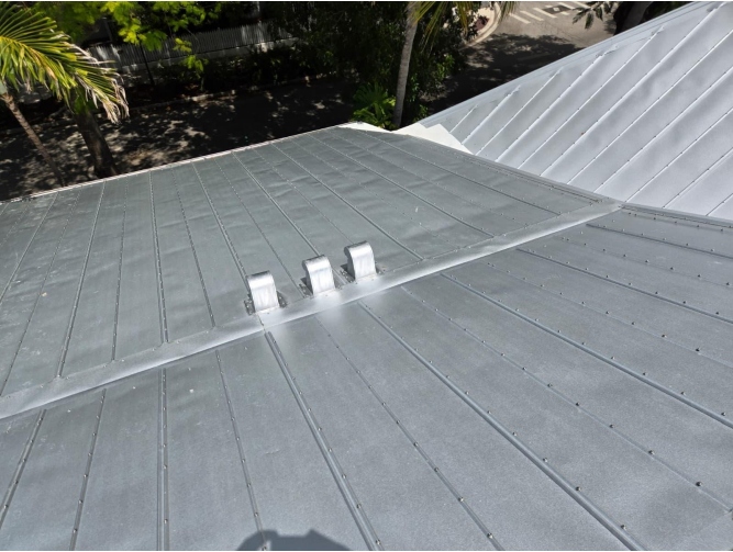
Metal roof photos
